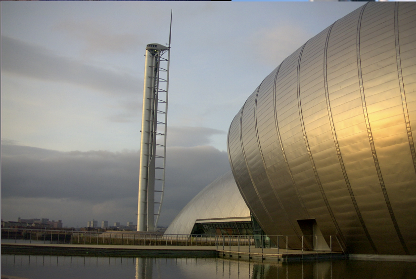
Tallest tower, Scotland, 360°, aerofoil, airplane wing, computer turn it in the wind to reduce wind resistance.
